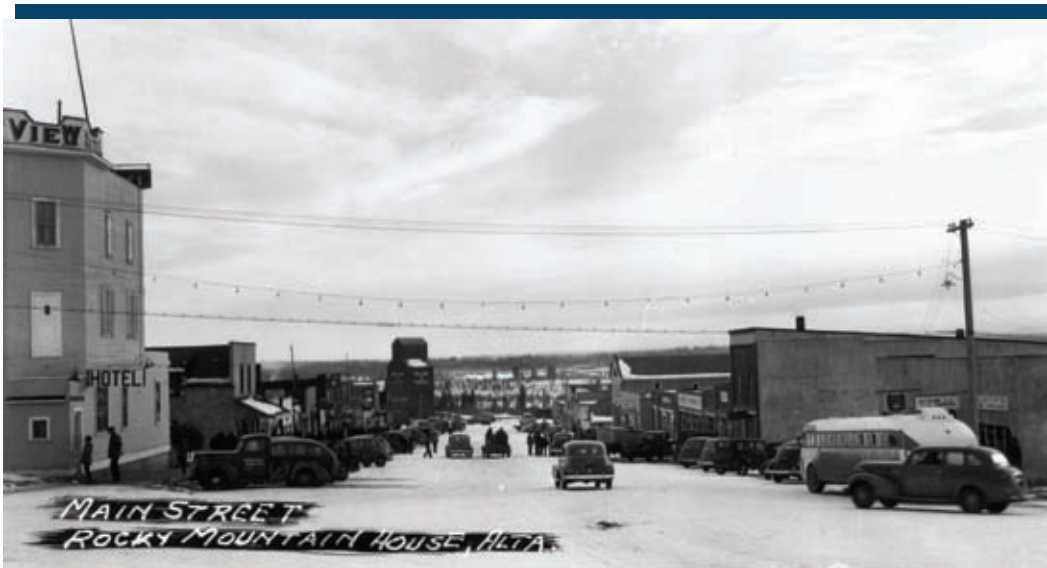
Looking South on Main Street, approximately 1950 Photo courtesy of Rocky Mountain House Museum
