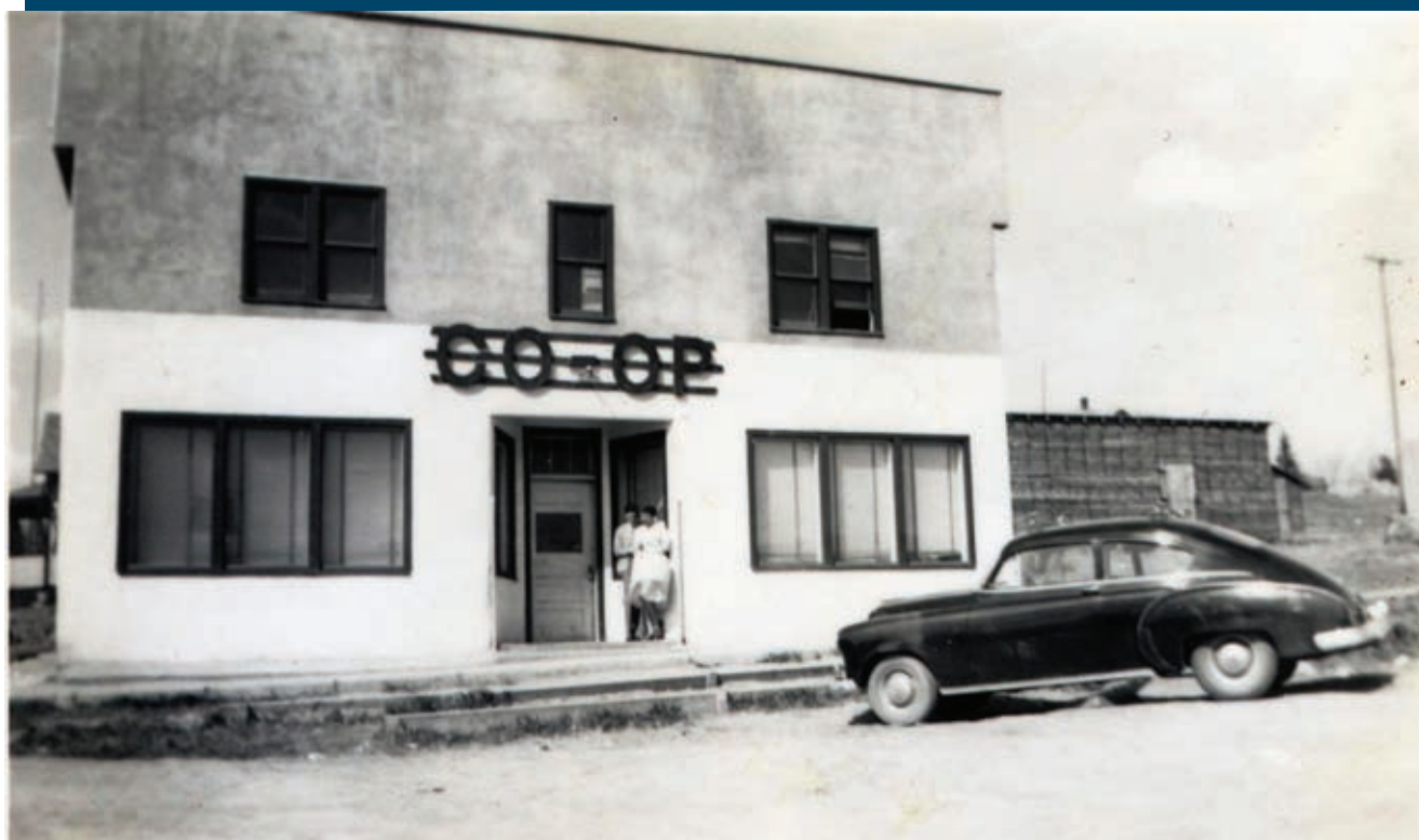
Old Co-op building on 50th Avenue, west of Main Street. Photo courtesy of Rocky Mountain House Co-op Association
